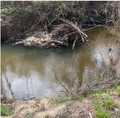
Trash collects in Walnut Creek near Dacian Road
