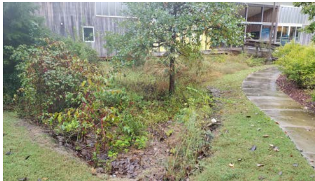
Image 7 & 8. Permeable pavement (top) and bioretention area (bottom) in front of the Walnut Creek Wetland Center. Photo Courtesy of Amin Davis.
